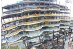
Central Steelwork; Hammersmith Road Lobby
