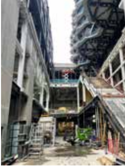
Hammersmith Road Escalator
